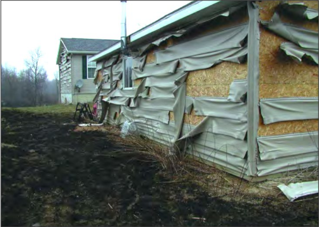
Figure 4. A wildfire in a grassy field melted the siding on this garage and home. (Courtesy of Michigan DNR.)
